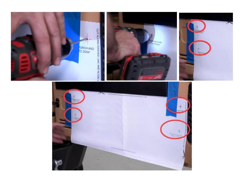
**Step 3:** Use the riveting nut gun with 6mm nut chuck to install the four riveting nuts.
