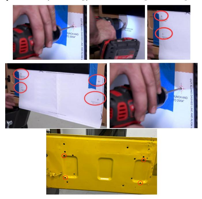
**Step 3:** Use the riveting nut gun with 6mm nut chuck to install the four riveting nuts
